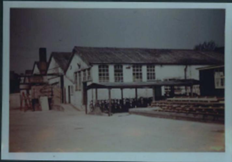
JOINERY SHEDS & SAW MILL
